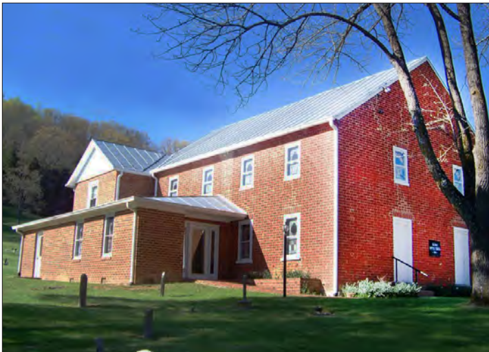
Neriah Baptist Church, in the South River community between Lexington and Buena Vista.
