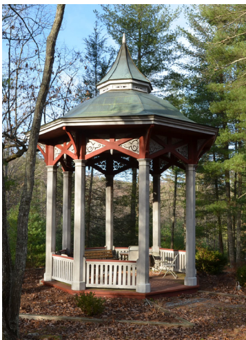
Gazebo at Jordan Alum Springs today. Photo by Arthur Bartenstein, from Architecture of Historic Rockbridge, Historic Lexington Foundation, 2015.
